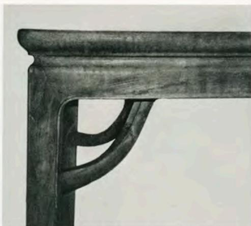
(Fig. 6f) Detail of a side table with giant's-arm braces
