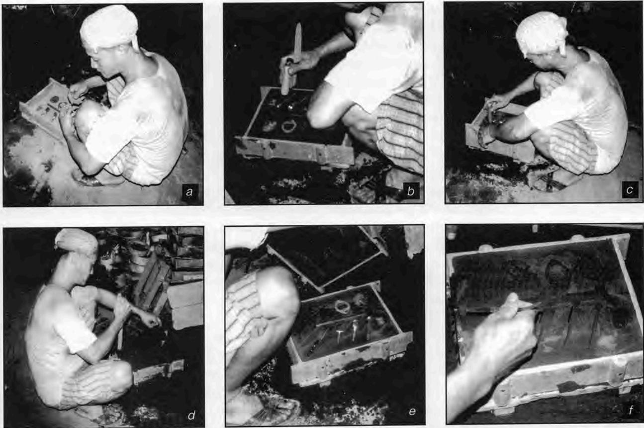
He also noted the use of various other tools, including tongs, hammers, and a steel scraper, whose sharp edges were presumably used to flatten the dimpled surfaces of hammered sheets of softer metals. The pump drill was also part of the tool kit, and was an indispensable aid in making small wares.
